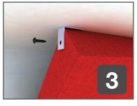
As per Section A and B, mark and fit 2 L Brackets at the far end of the trap and fix into the MDF edging of the trap with 4 'pan head' wood screws.
